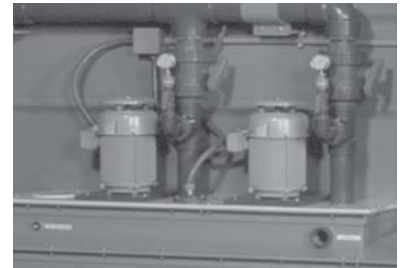
Dual Redundant Pumps
